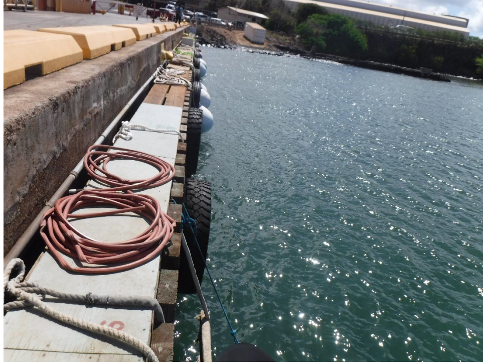
Photo 5: Fender System and Waterline
